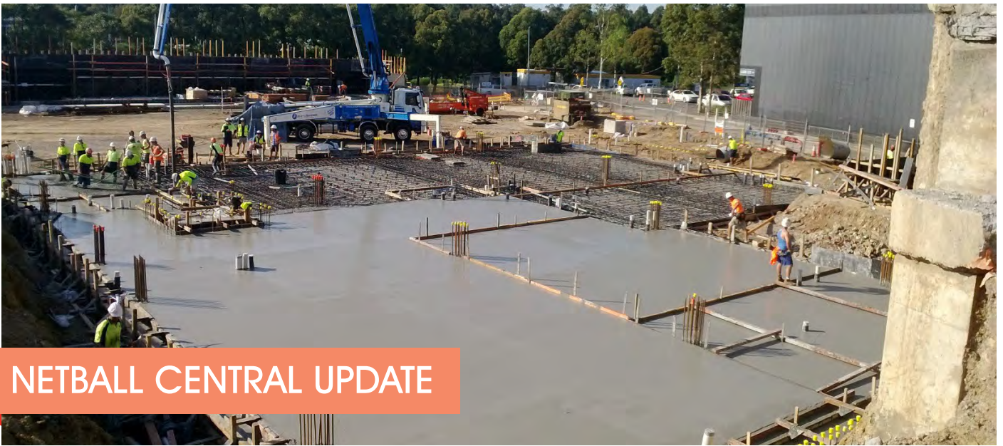
Laying the foundations of the Netball Central project site at Sydney Olympic Park
