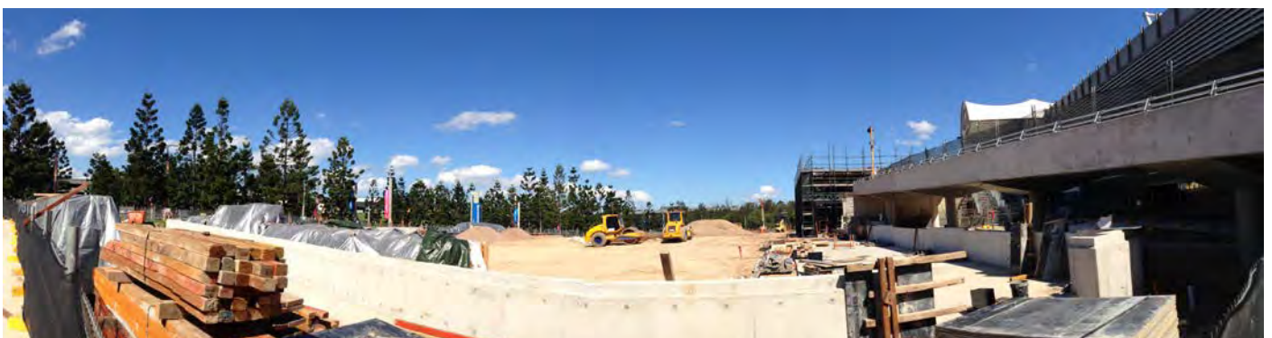
Netball Central under construction
