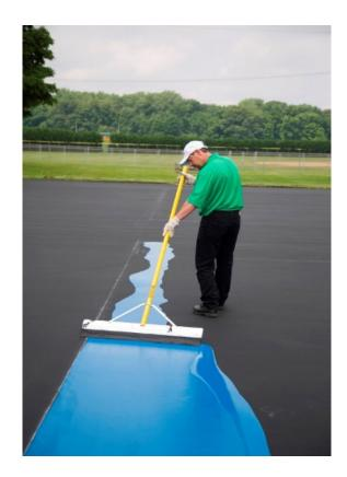
The acrylic coating provides appropriate surface texture for fast modern netball. It reduces abrasions, it is less fatiguing with sound traction for players.
