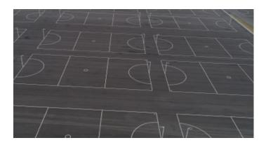
Asphalt is not a structural product. It has compressive strength but it does not have significant tensile strength. It relies on a solidly, well compacted, well drained sub base to maintain its surface profile. Having compressive strength but low tensile strength means it will not depress or rise unless there is movement in the sub-base. Therefore, it is very important to have a well-engineered sub pavement.
